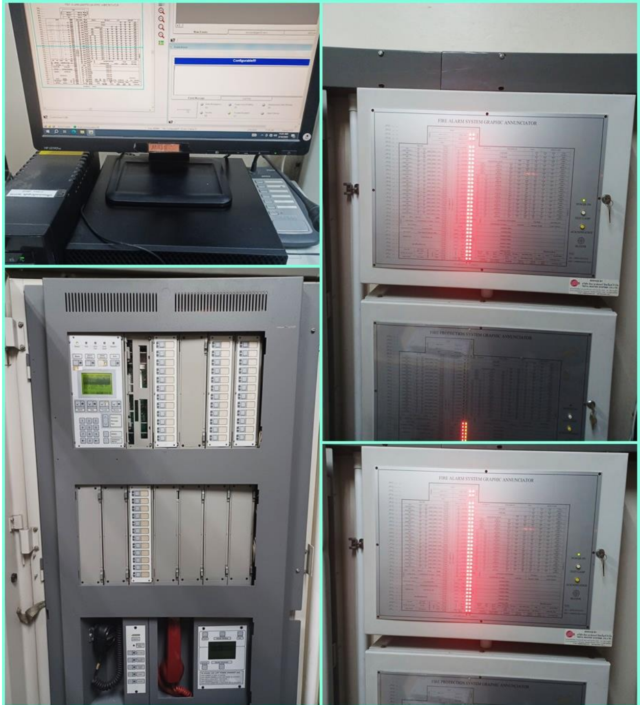
រូប​ភាព 12.34 Fire Alarm Control Panel : FCP
